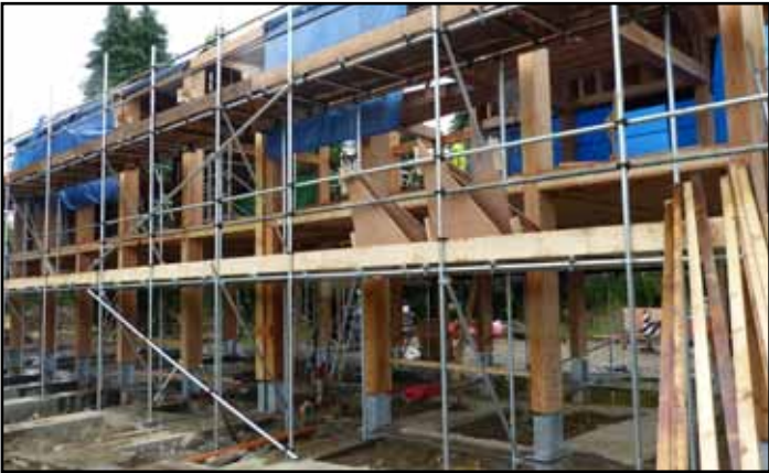
Figure 10: Ty Unnos portal frames erected at Blaengors, Carmarthenshire (image: courtesy of Coed Cymru)
