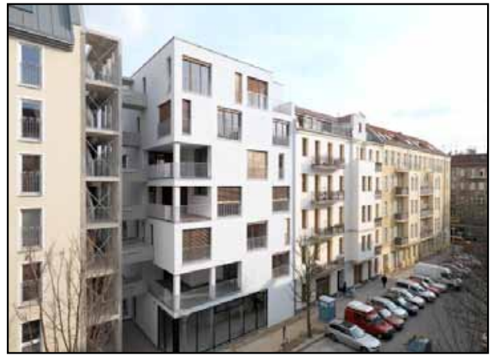
Figure 30: The seven storey Brettstapel e3 apartment block in Berlin (image: courtesy of Bernd Borchardt and Kaden + Klingbeil)
