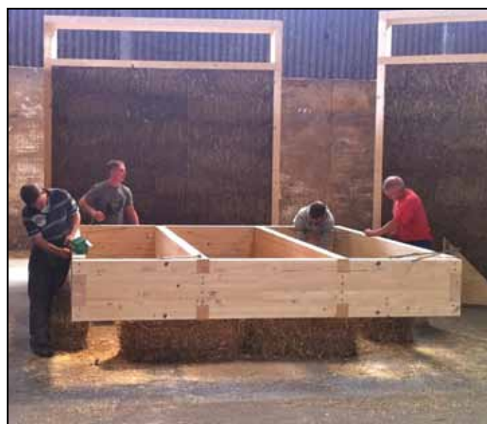
Figure 26: A Modcell cassette being fabricated in a 'flying factory' (image: courtesy of Craig White)
