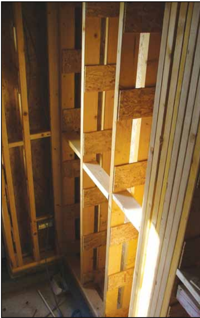
Figure 17: Twin-wall construction with OSB gussets prior to filling with insulant (image: courtesy of Williams Homes)
