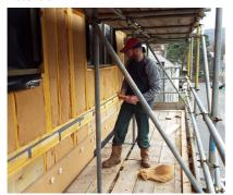
Company Director Gary Newman on site installing plant fibre insulation on a low carbon Williams Homes timber frame housing project
